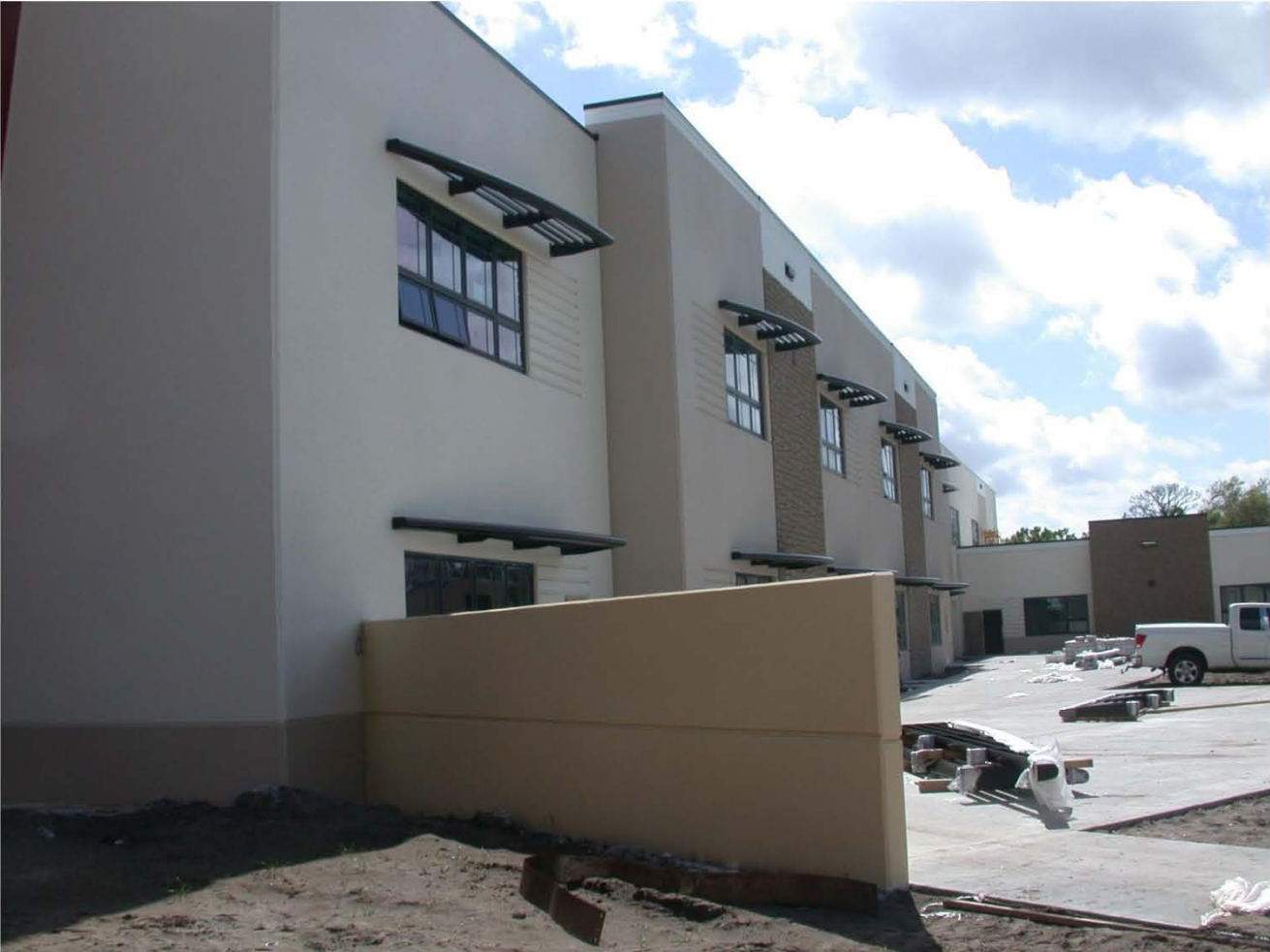
Vero Beach Elementary: Exterior of Building 2 Facing West
